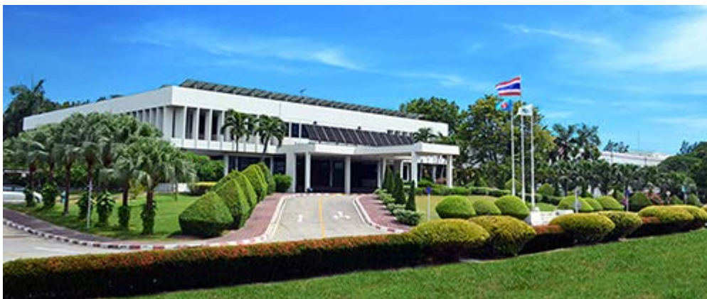
SIAM COMPRESSOR INDUSTRY CO., LTD.
