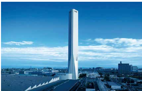
SOLAÉ elevator testing tower
